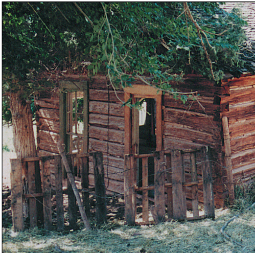
The house and its corner joints in 1999. Author photo
